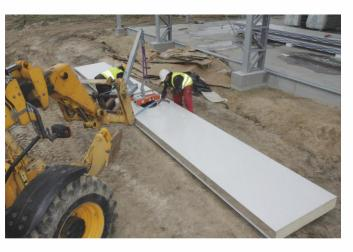
$\bigcirc$  **1b.** lifting the machine together with panel
