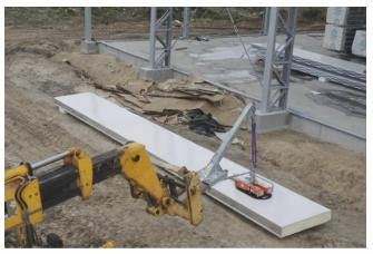
○ 3b. lifting the machine together with panel
