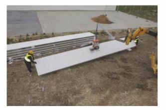
Damage free installation of sandwich panels with VIAVAC vacuum lifters
