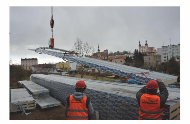
Damage free installation of sandwich panels with VIAVAC vacuum lifters
