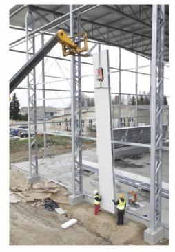
$\bigcirc$  3a. situating the machine and its attachment to the panel
