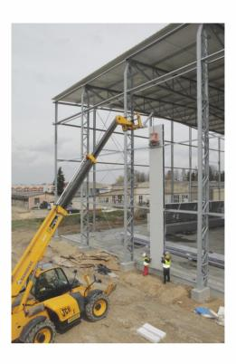
D Damage free installation of sandwich panels with VIAVAC vacuum lifters
