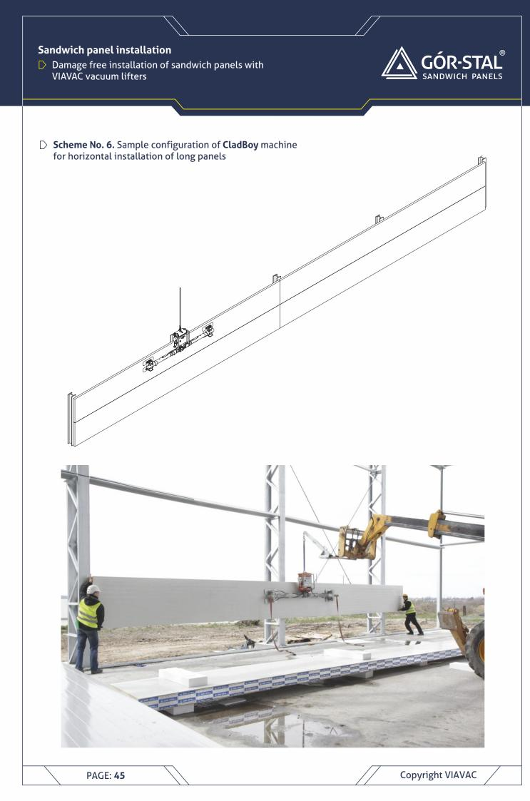
D Damage free installation of sandwich panels with VIAVAC vacuum lifters
