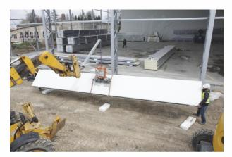
$\bigcirc$  2d. installation of panel on the wall and detachment of the machine
