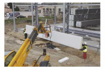
[ig> 1d. installation of panel on the wall and detachment of the machine
